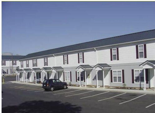
This eight-residential-unit building is typical of a small MDU in that the entryway to each unit is external to the structure and the building does not exceed three floor levels in height.
