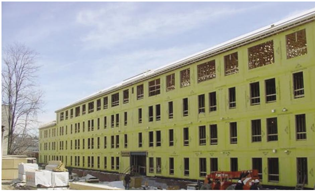
This medium-size MDU under construction provides an opportunity for a greenfield FTTM installation.
