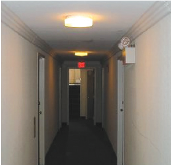
Figure 4.6 – Raceway in the Form of Decorative Crown Molding | Photo NS124
