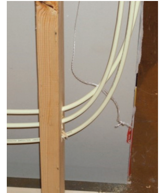
Figure 4.3 – Sweeping Bends of Microduct in Joist | Photo NS157
