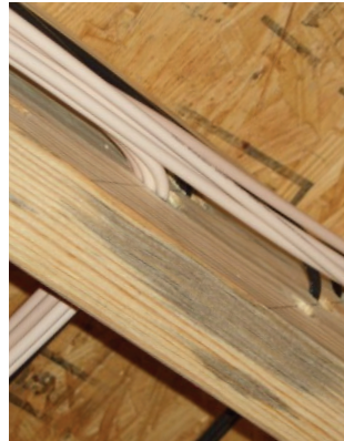
Figure 4.2 – ClearCurve Rugged Drop Cable Installed Through Joist | Photo NS159
