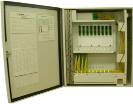
Fiber Distribution Hub
